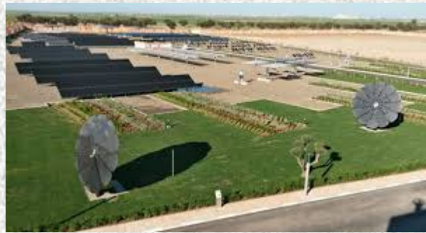
Station solaire Noor I Ouarzazate
